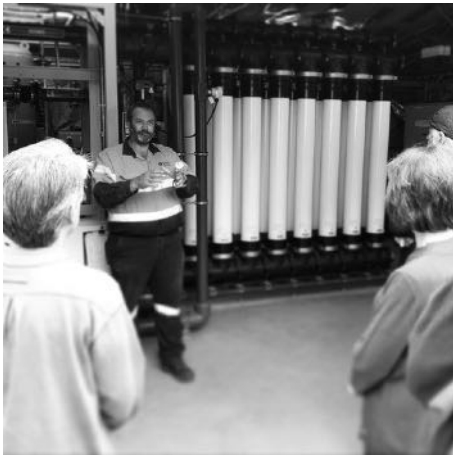
Coliban Water Plant There's half a hectare of filtration surface in those filters! Picture: Nat Cursio
